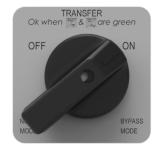
Warning: When the system is in by-pass, the load is subjected to AC main disturbances.
